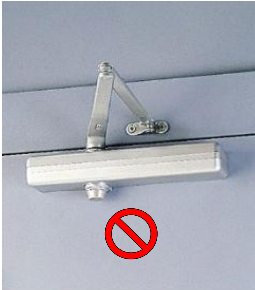
Figure k: Unsightly lever arm door closer
