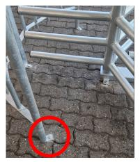
Then continue mounting the screen to the substrate by securing the remaining drill holes with a chemical anchor. Make sure these are in a straight line.
